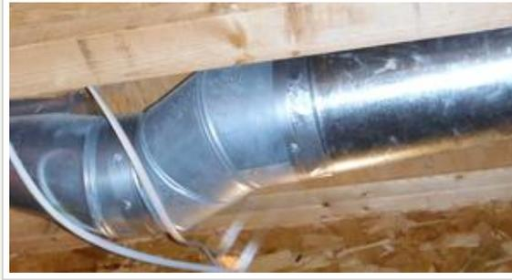
Duct tape is not a proper seal for duct work. Mastic or metal tape should be used.
